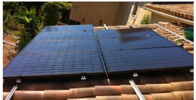
*Figure 1 : installation on K2 overlay system*
